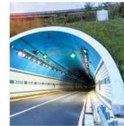
BORIVALI - THANE TUNNEL
