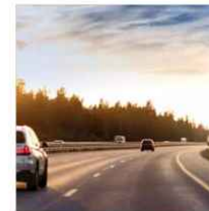
CENTRAL PARK ROAD LINKING KOLSHET & BHIWANDI
