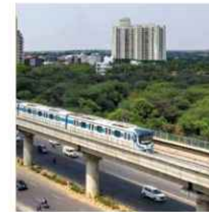
MUMBAI METRO LINE 5
